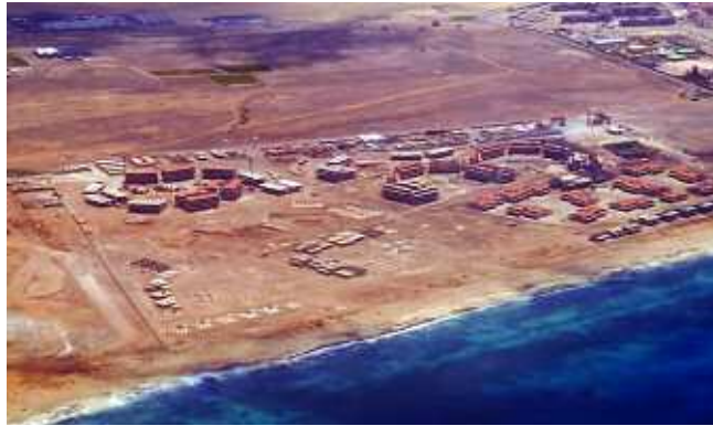
A number of structures are now complete across the site.
