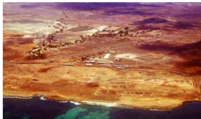
The scale of the project can be seen from its front-line beach position.
