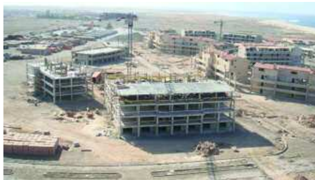
Building is well underway.
